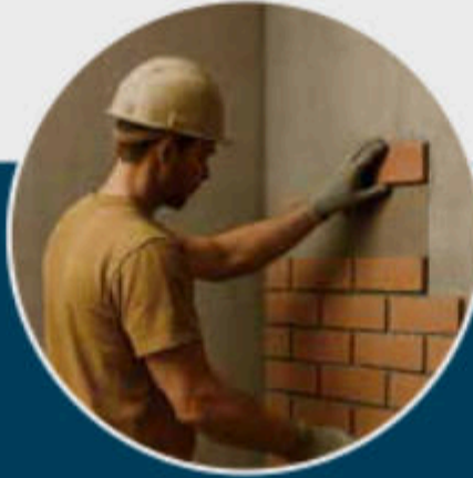
3. Installation on Surface
